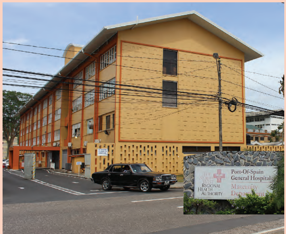
Port of Spain General Hospital Maternity Department.
